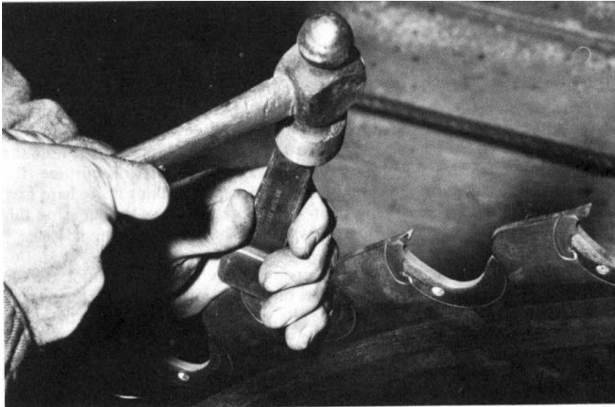
Figure 42. – Proper swaging requires positioning, holding, and striking the swage correctly.
